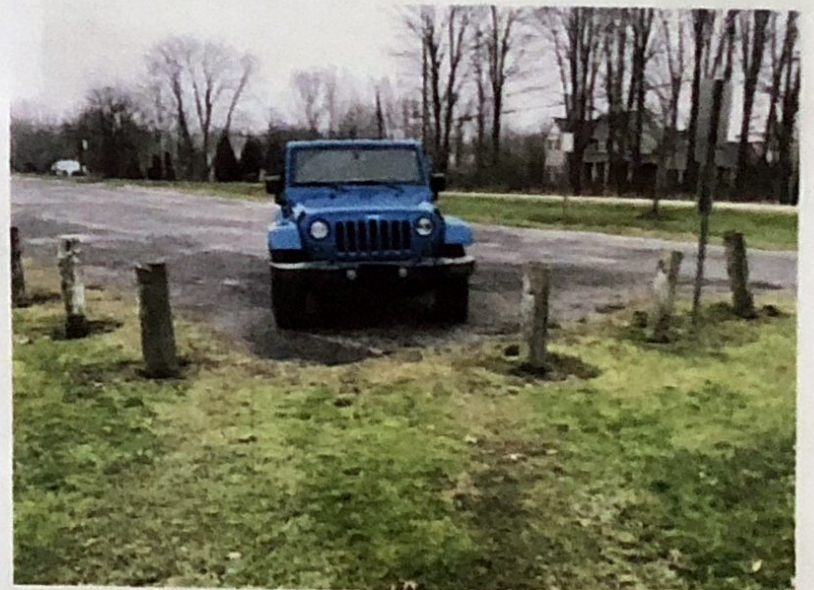
Below: Can see the opening is wide enough for a vehicle to drive through.
